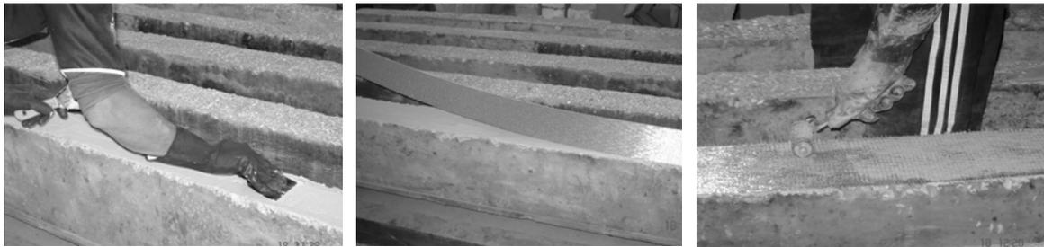
Figure 5. Typical application procedures of SRP
